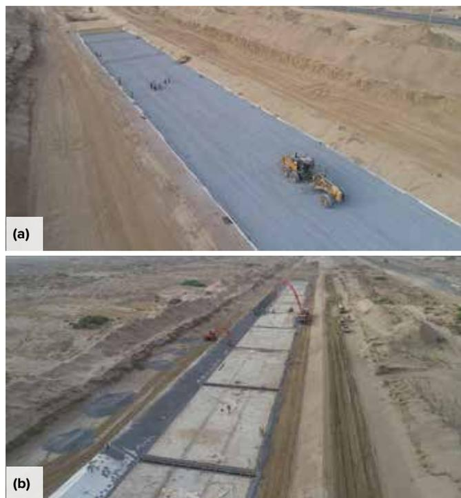
Fig. 5: Placement of the drainage layer: (a) for the base slab; and (b) for the sloped sides. The drainage layer for each of the sloped sides of the channel was placed after completion of the blinding layer for the base
